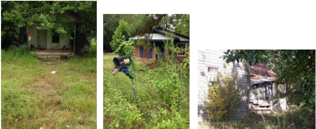
Figure 13: Deteriorated or dilapidated homes in South Hartsville
